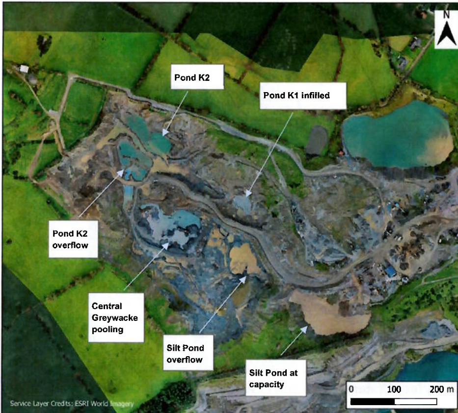
Figure 6-7 - Site Aerial with Surface Water in October 2023 (Images from site survey)
